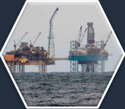
Offshore Gas Processing Facility
