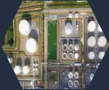
Tank farms (Blending automation)
